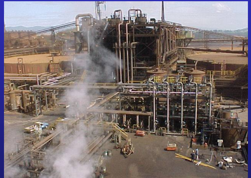
Refinery Heat exchanger
