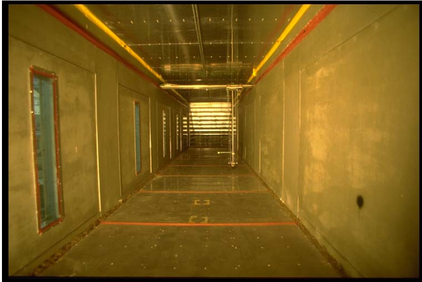
Interior of the tunnel
